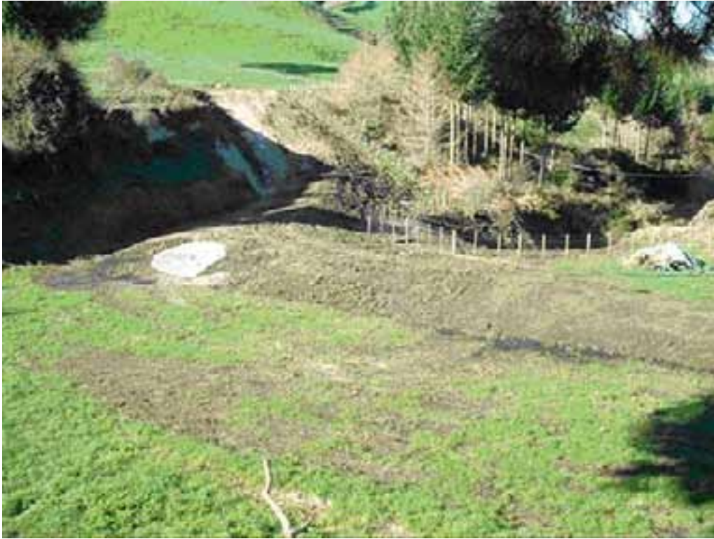
Photo 14: Newly created detention bund with concrete outlet.
