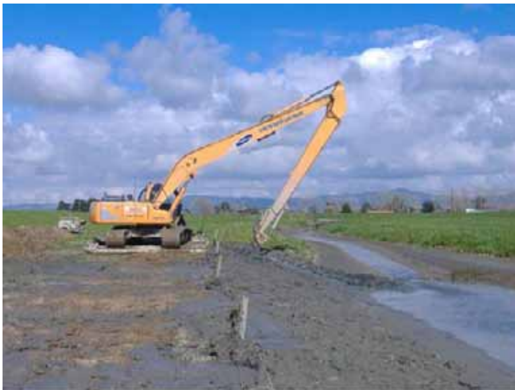
Photo 22: Silt removal.
