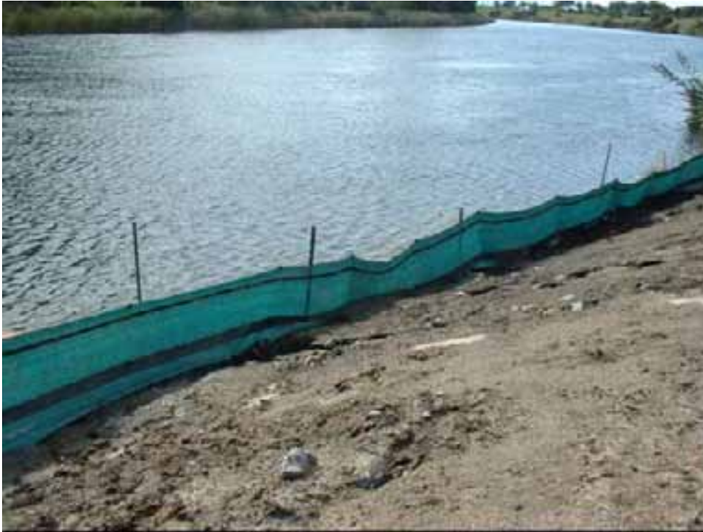
Photo 24: An example of a silt fence built to reduce sediment entering the water.
