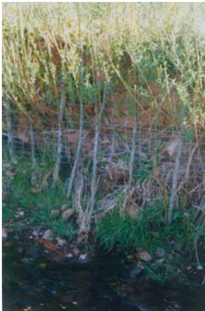
Photo 8: Shrub willow tied into bank for erosion control.
