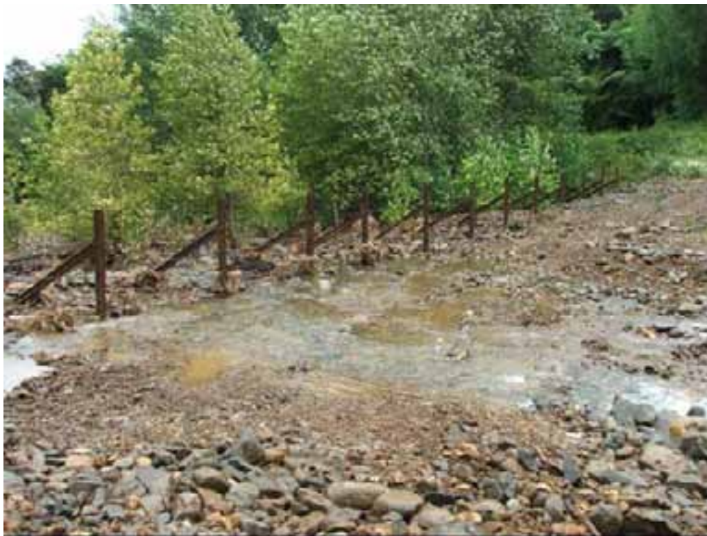
Photo 15: Debris trap across a stream.
