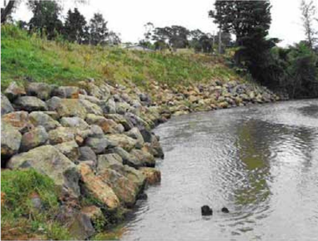
Photo 11: Rock riprap used to stabilise an eroding river bank.
