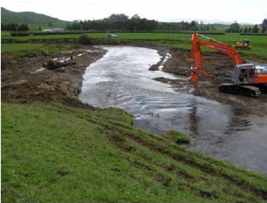
Photo 18: Excavator working from dry ground re-aligns the river.
