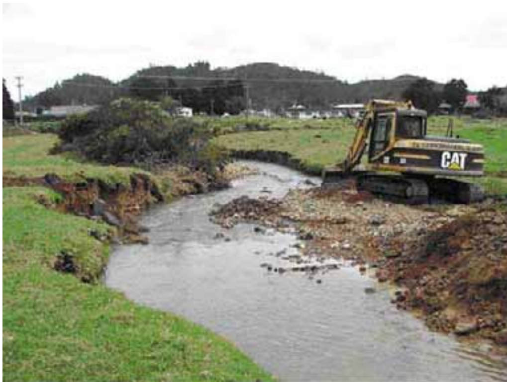
Photo 16: Movement of gravel from the right bank to alleviate erosion on the left bank.
