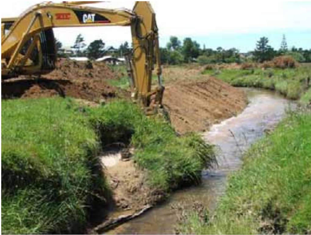
Photo 20: Excavator undertaking bank battering.
