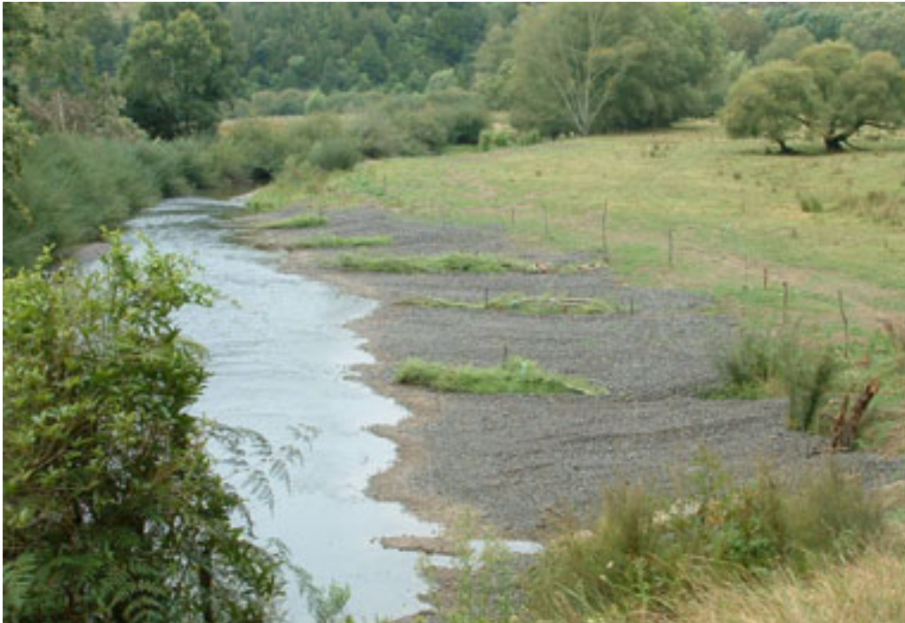
Photo 1: Newly constructed groynes on the right bank.
