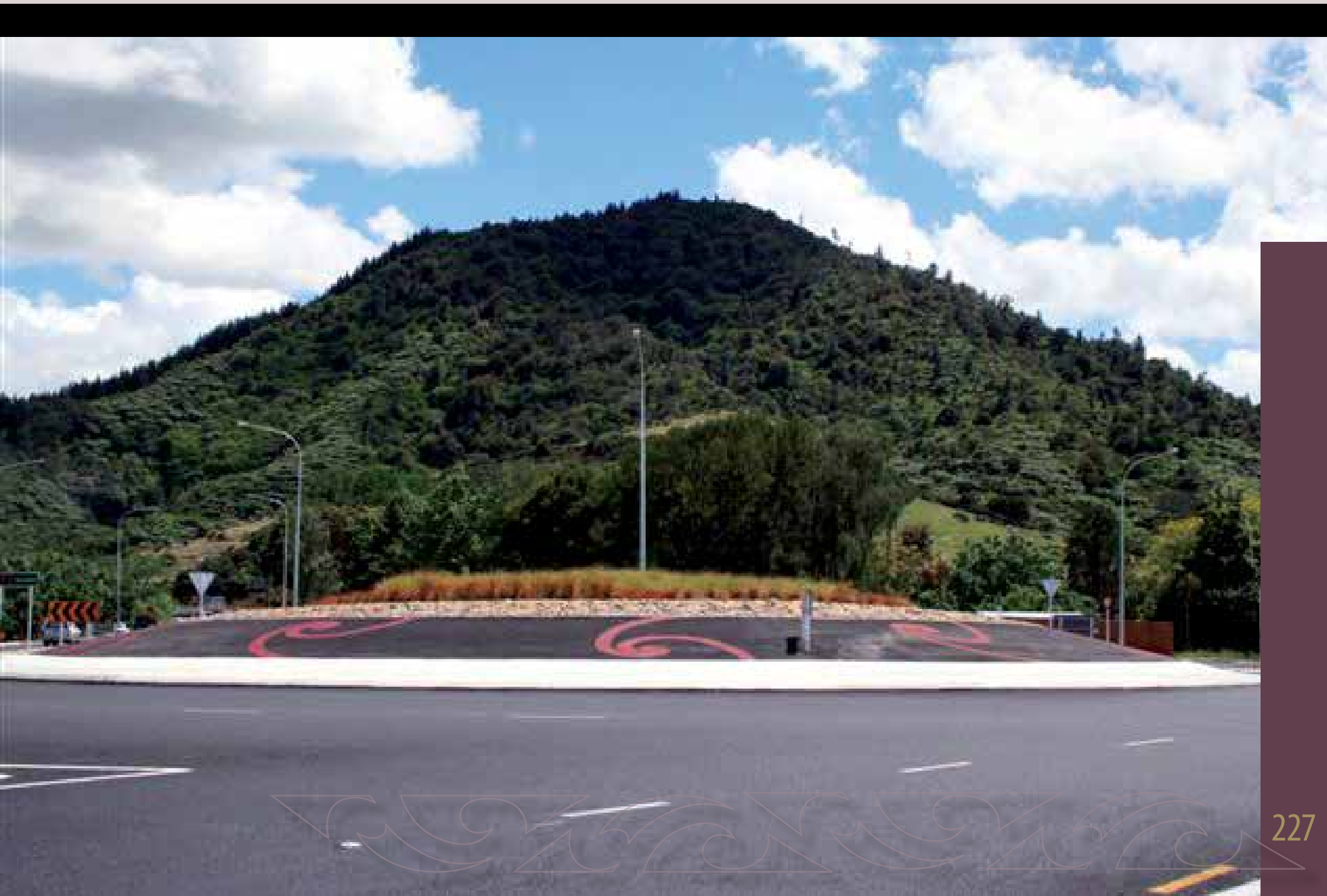
Taupiri Roundabout, Waikato Expressway
