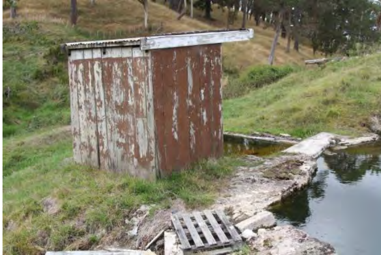
The larger geothermal pool at Horohoro. Note the changing room near the outlet of the pool. (February 2014)
