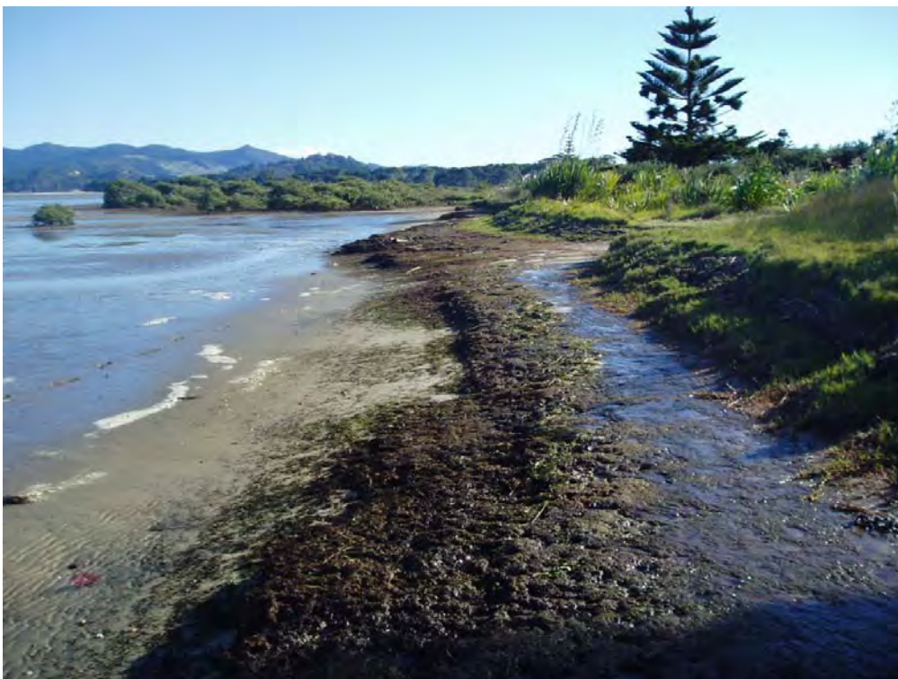
Figure 7: The eroding shoreline north west of the Matarangi boat ramp.
