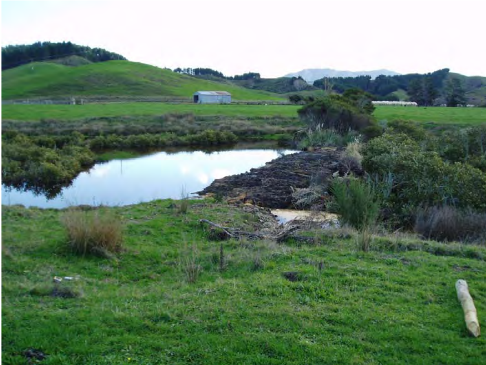
Figure 42: An earth dam prevents the natural flow of salt water upstream.
