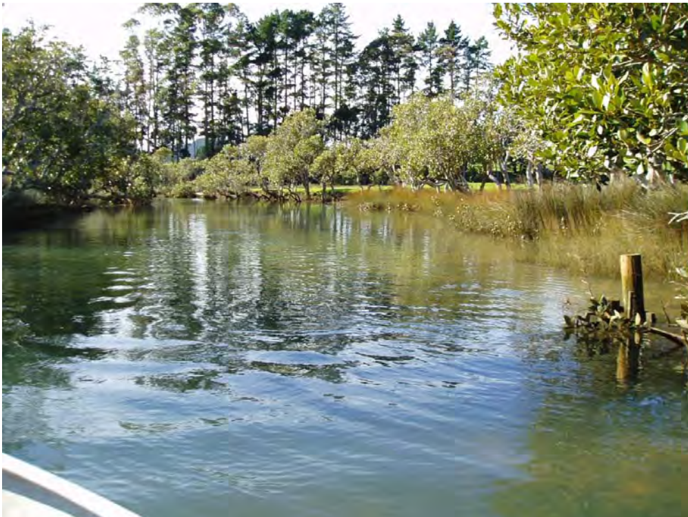
Figure 23: Another view of unprotected banks of the Otanguru Stream (TRB).
