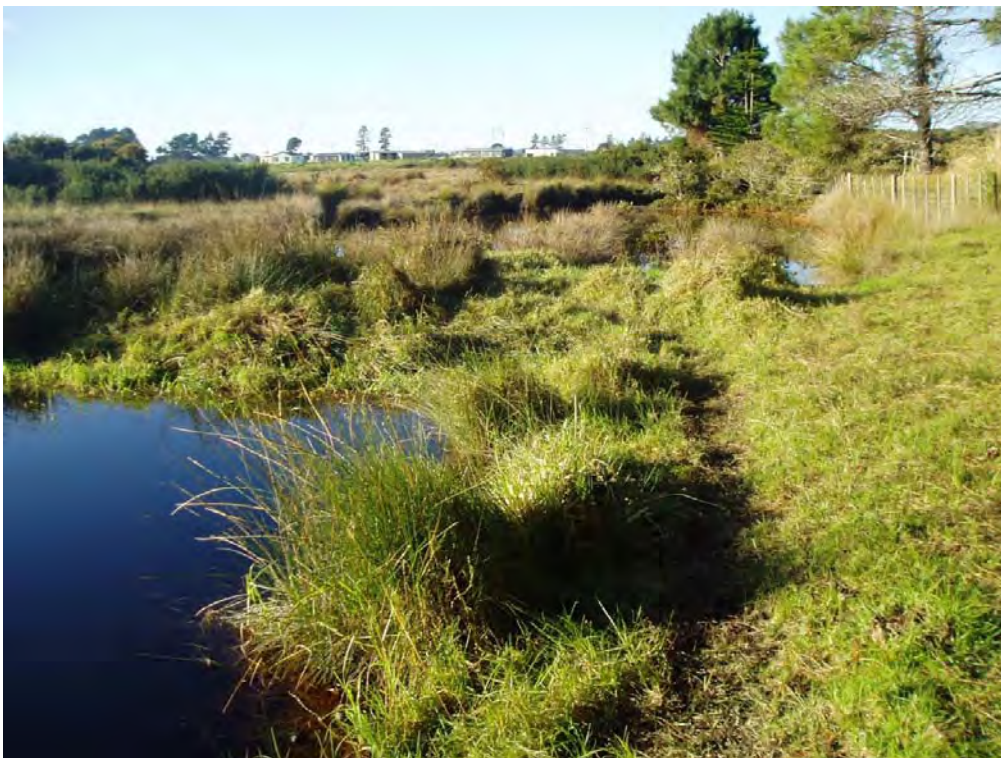
Figure 9: This small embayment of the harbour has been bunded and drained resulting in markedly different water levels in the ponding areas either side of the bund.
