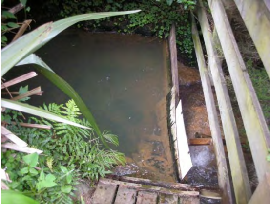
Figure 9: The North Pool at Golden Springs Motel
