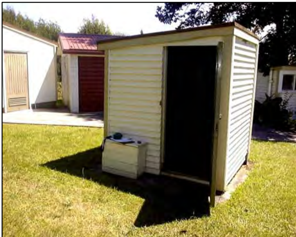
501. Location of Pump shed
