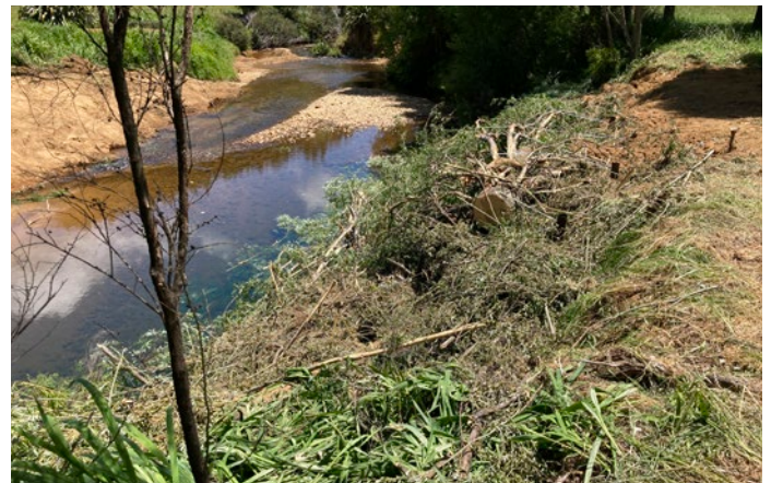
Tree layering along the Kaimarama River helps protect the bank from erosion.
