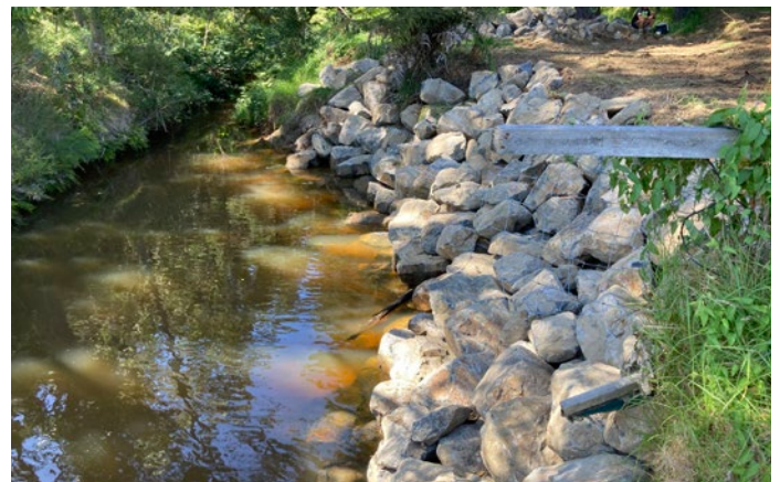
A rock revetment put in to protect a section of the Wahitapu Stream bank from eroding.
