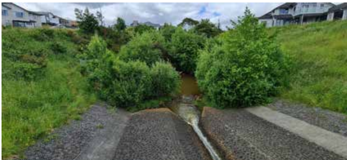
Photograph 3.1: Vegetation observed around the stilling basin downstream of Magellan Lake showing grey willow growing around the stilling basin.
