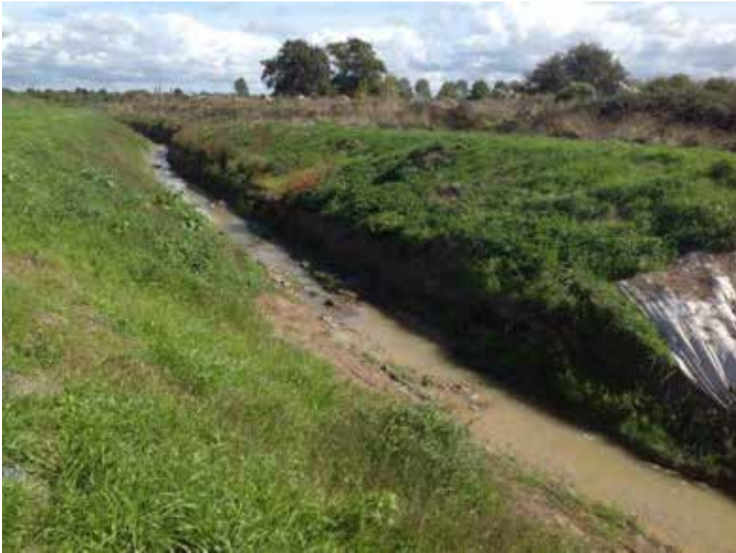
Plate 3: Established swales upstream of Resolution Drive.
