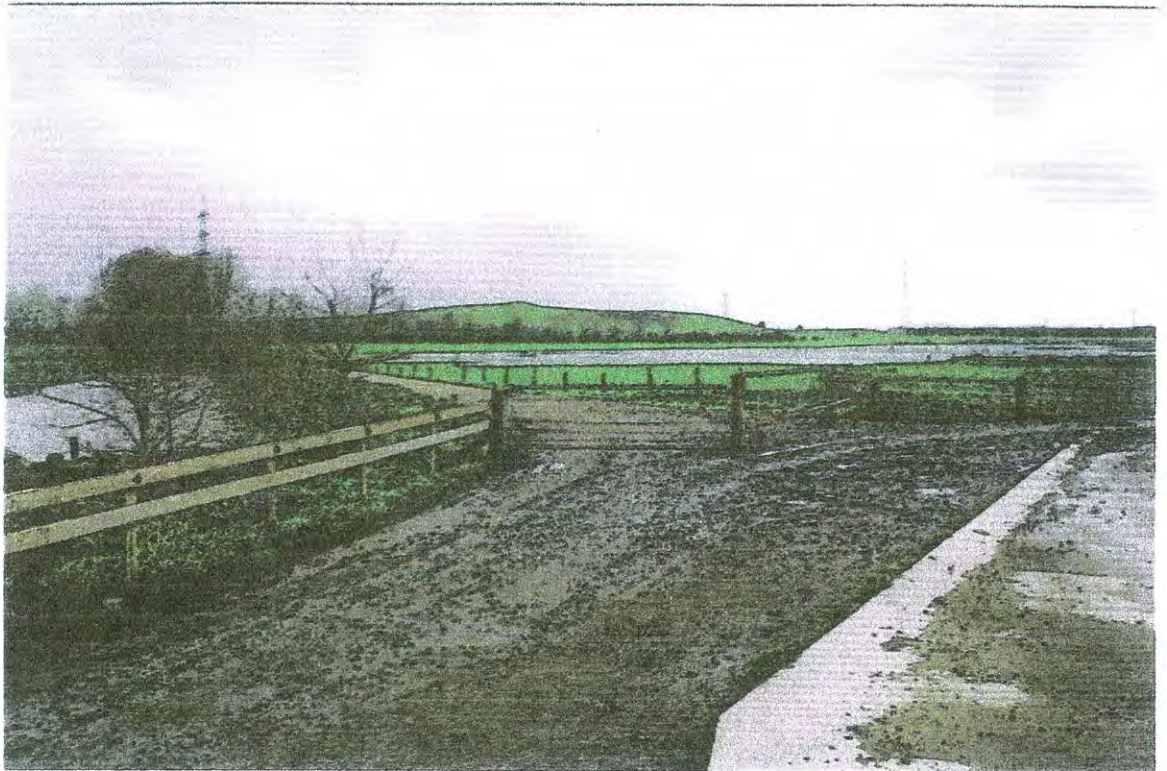
WUA built step bank with drain elements.
