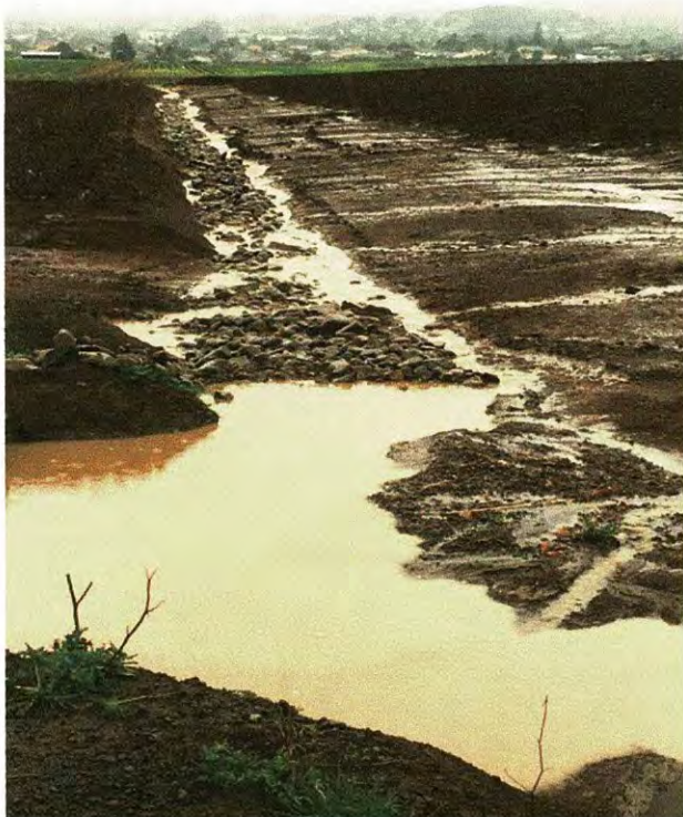
River rock mitigating erosion. Home Block
