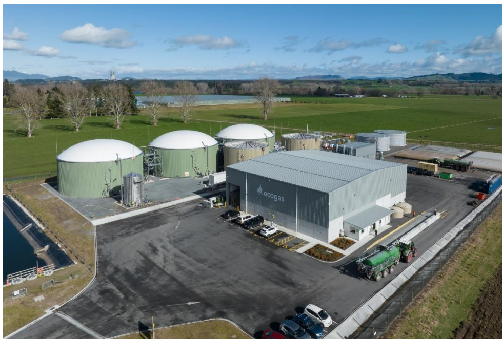
Figure 3-14 Ecogas facility, Reporoa (Ecogas N.D.)
